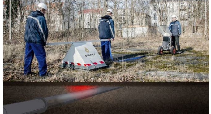
EMPIT-Crew during inspection
