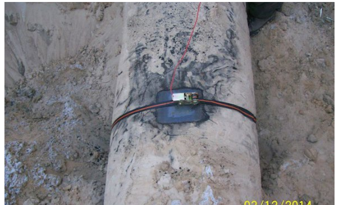
Connection through dug hole
